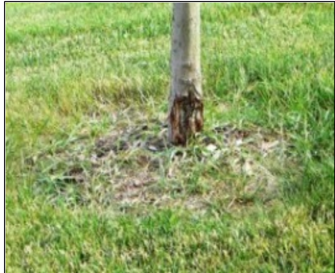
Mechanical trunk damage
