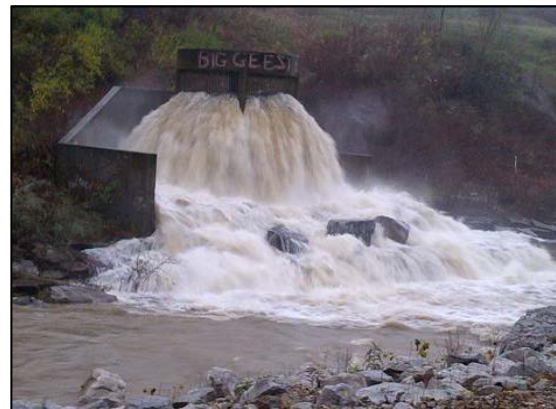
Combined sewer overflow after a rain event.
