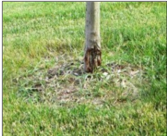
Mechanical trunk damage
